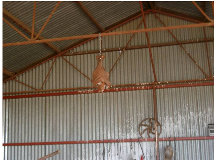
Figure 4. Terracotta bat back in place.
